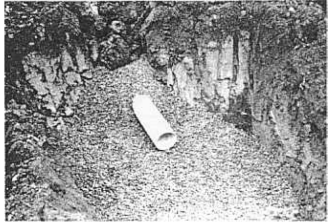
FIGURE 1: Tested in the field under difficult conditions, the use of lightweight aggregate as bedding for a sewer line proved successful.
